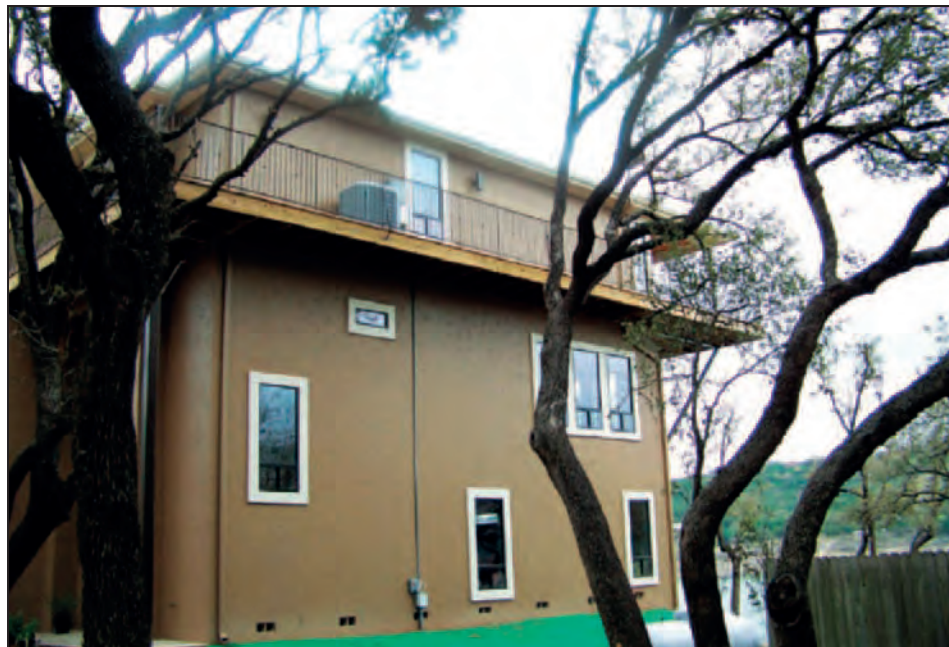
Figure 2-24. Two-story enclosure SOURCE: FEMA P-499 2010
