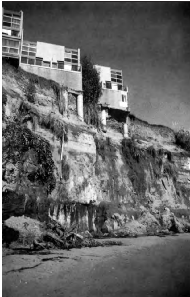
Figure 3-37. Bluff failure by a combination of marine, terrestrial, and seismic processes led to progressive undercutting of blufftop apartments at Capitola, CA, where six of the units were demolished after the 1989 Loma Prieta earthquake
