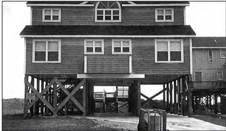
Figure 10-10. Diagonal bracing using dimensional lumber
