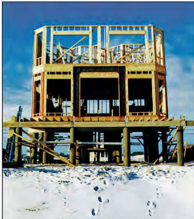
Figure 9-25. Steel moment frame with large opening
