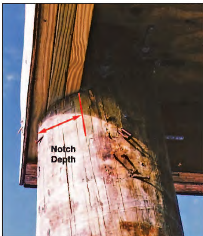
Figure 13-4. Properly notched pile; outer member of this three-member beam supported by the through-bolt rather than the beam seat
