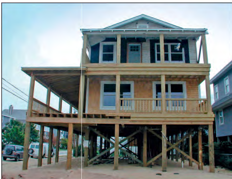
Figure 15-9. Home elevated on piles
