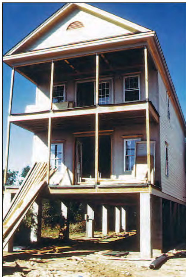
Figure 13-6. Open masonry foundation
