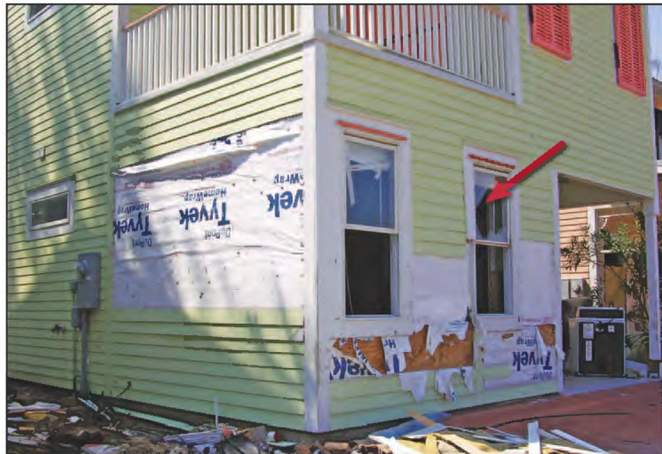
Figure 11-16. Blown-off fiber cement siding; broken window (arrow). Estimated wind speed: 125 mph. Hurricane Katrina (Mississippi, 2006)
