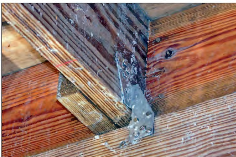
Figure 9-17. Metal joist-to-beam connector
